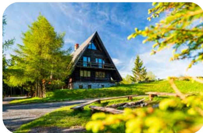
PTTK Mountain Hut at the Okraj Pass (Photo: R. Kotylak)
